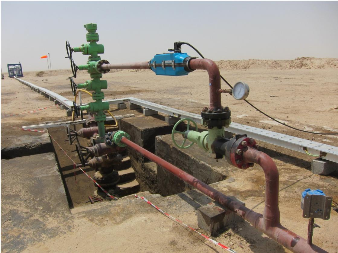
**Figure 20: SONAR meter installed on an ESP Well in Middle East**
