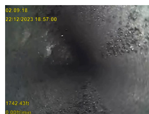
After CoilHose Intervention
