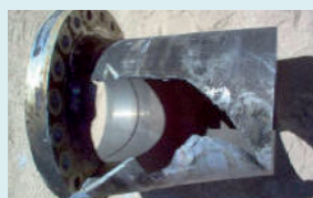
Aluminium component (corroded by mercury), which failed, leading to a fire
