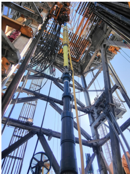
View of the Fast Response System (yellow) with the Lower Landing String (blue) in the rig's derrick
