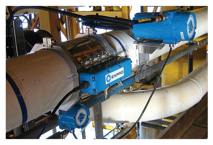
We utilise clamp-on sonar-based meters and innovative multiphase flow interpretation techniques to provide accurate and reliable flow measurement with no process interruption.
